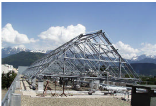
Figure 3.1: Photo of the project - Surieux. View from the ridge roof.
