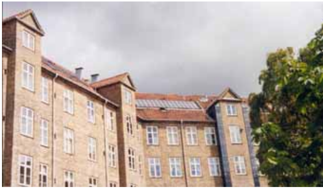
PV in old roof in housing block Trekanten at Frederiksberg
