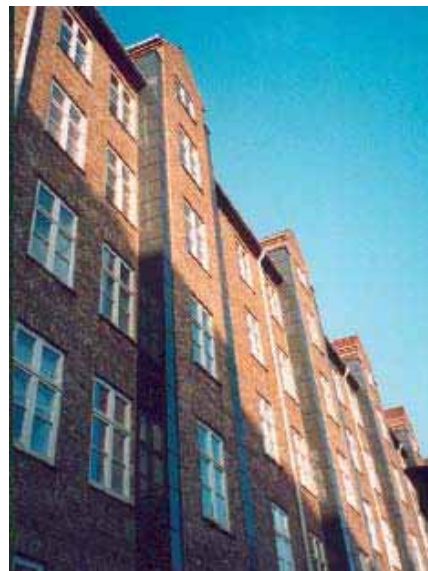
Figure 15. The ventilation towers, Lineagården, Frederiksberg
