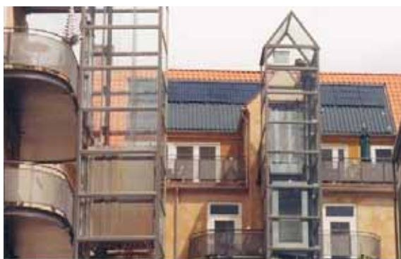
Housing project Lauritz Sørensensgård, Frederiksberg in Copenhagen. PV placed on top of ventilated Canadian solar wall.
