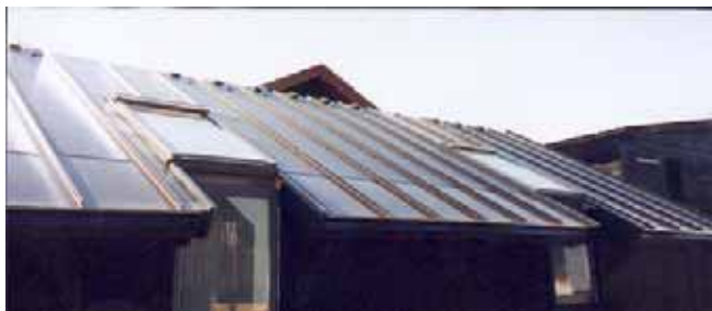
CO 2 neutral test house. PV integrated in metallic roof.
