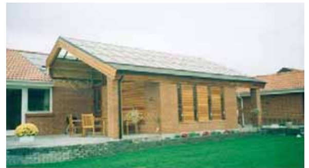
PV panels on family house
