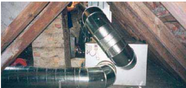
Figure 16. Counter flow heat recovery unit.
