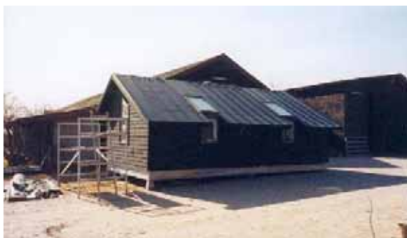
CO 2 neutral test house.
