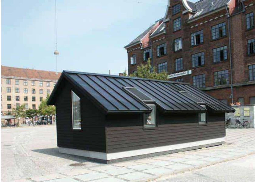
Figure 10. Exhibition of CO 2 neutral test house at Toftegårds Plads in Copenhagen (until end of 2003).
