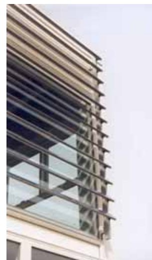
PV shading systems (ALU-PV) at students house in Herning
