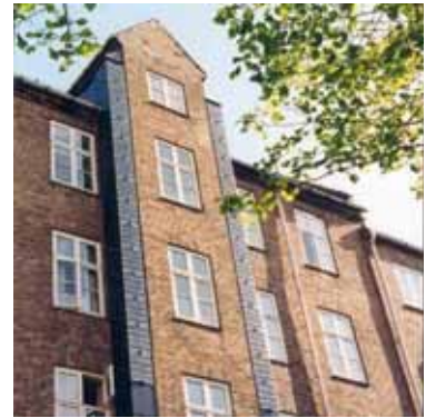
Trekanten, PV panels integrated together with solar ventilation towers which have built in duct work for heat recovery ventilation systems
