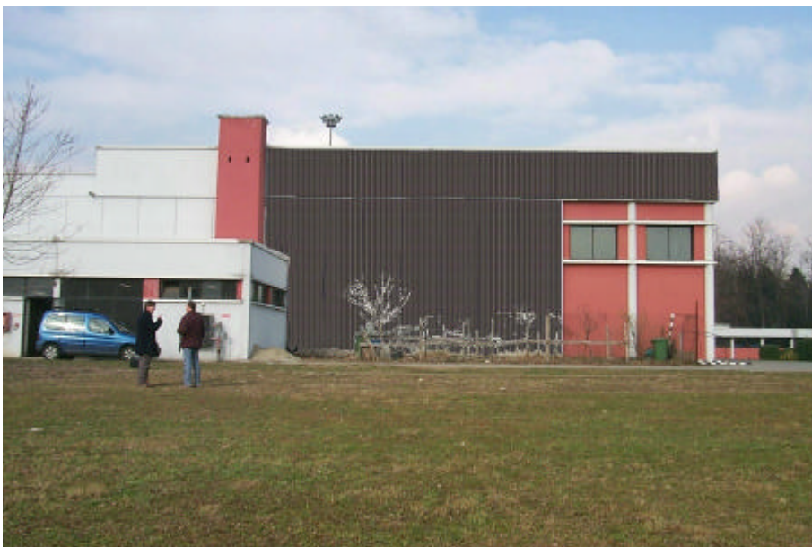
Pioltello: Solarwall air solar collectors on the south facades
