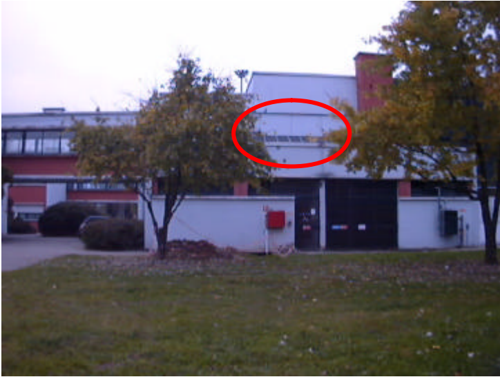
Pioltello school centre: PV modules on the roof of the thermal central plant.
