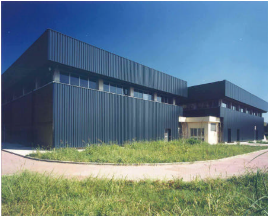
Cernusco sul Naviglio: Solarwall air solar collectors on the south facades
