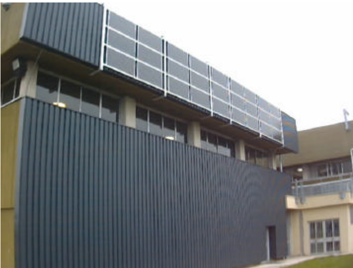
Cernusco sul Naviglio school centre: PV modules mounted on the Solarwall collectors
