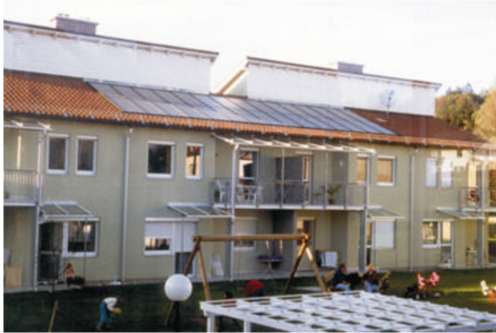
Fig. 8: Multifamily building with 8 dwellings and a solar plant consisting of 60 m 2 collector area and 2,4 m 3 storage tank only for domestic hot water preparation
