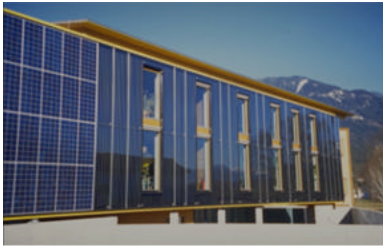
Fig. 7: Facade integrated collector, DHW preparation for showers and direct floor heating in winter time with lowest temperatures for high efficiency (Source: DOMA)
