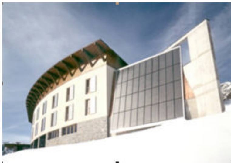
Fig. 6: Hotel Bielerhöhe / Sylvretta (28 beds, 60 m 2 collector area, 14 m 3 tank in tank system including 900 ltr DHW-tank)
