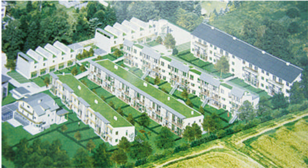
Fig. 12: Large-scale solar heating system, Salzburg Gneis-Moos (400 m 2 collector area, 100 m 3 water tank, appr. 60 flats)
