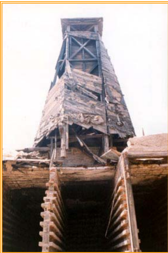
CHIMNEY PRIOR RENOVATION
