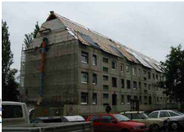
Placing the insulation.
