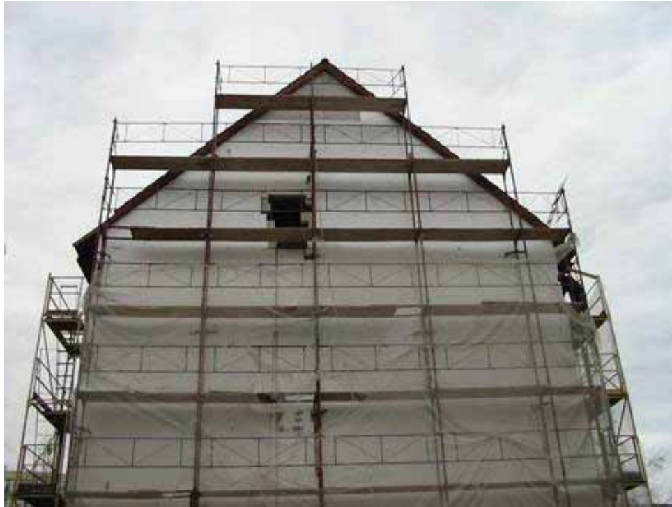
Placing the insulation.
