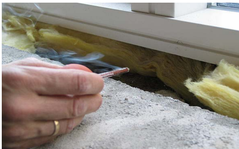
Figure 2: Example of test of white smoke movement regarding airtightness.
