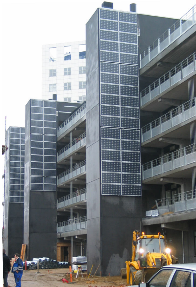
Figure 3. 200 m 2 PV modules have been mounted on the towers in the housing project Dalgas- parken in Herning with 72 apartments.
